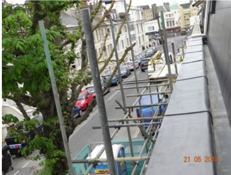
Fig 3: Neoprene Jointing
