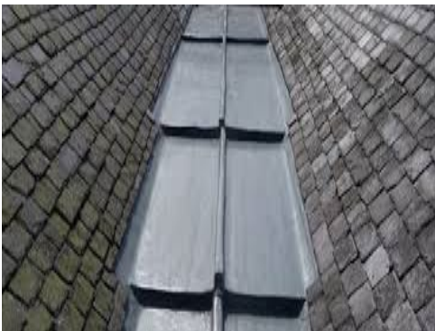
Fig 1: Traditional Stepped Detail
